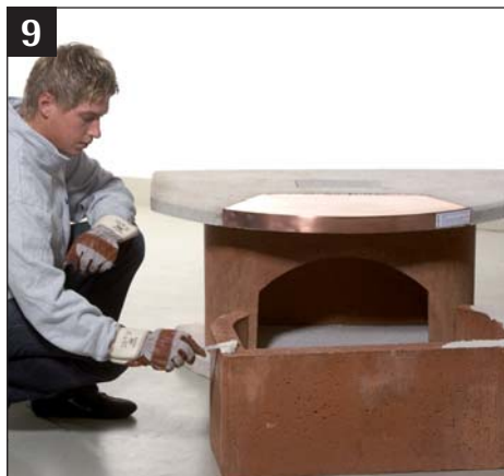
Apply mortar on the lower edge of the fire box
