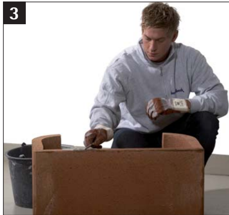
Apply mortar on the lower edge of the base and wood storage
