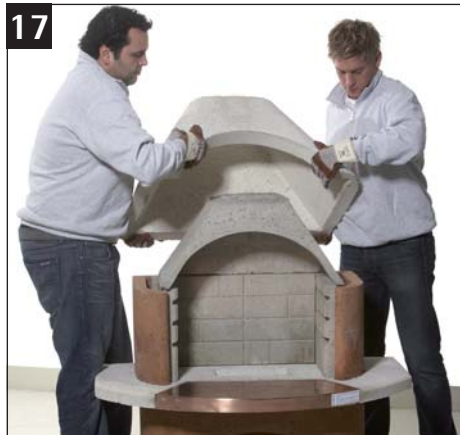
17 Mount concrete hood flush to the back of the firebox
