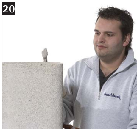
20 Apply mortar on the upper edge of the chimney extension
