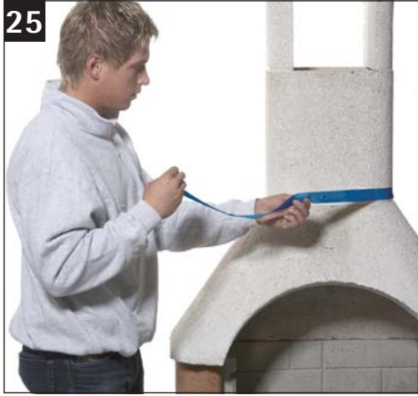
Remove the tape after the mortar sets.
