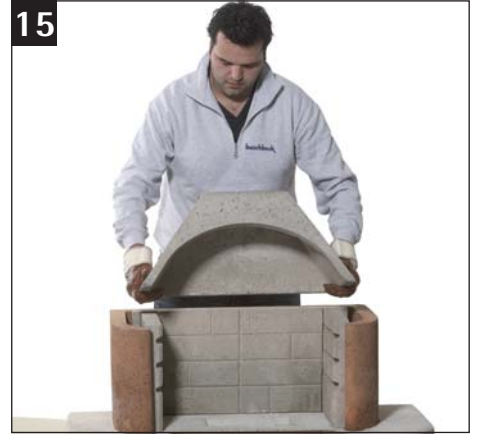
15 Mount firebox hood. The rear should line up with the inside rear firebox wall.
